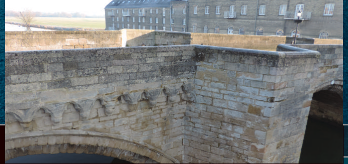
The bridge over the Great Ouse at Huntingdon. During the Civil War, a span was removed and replaced by a drawbridge. The span was later replaced but as this view shows, is different from the original (closest to the camera). Image by David Flintham
