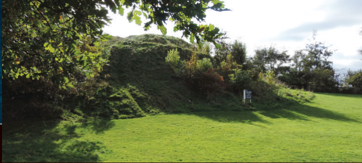
Cambridge Castle was incorporated into the city's fortifications in 1643. This view shows the remains of the motte, and the edge of the east bastion to the left. Image by David Flintham
